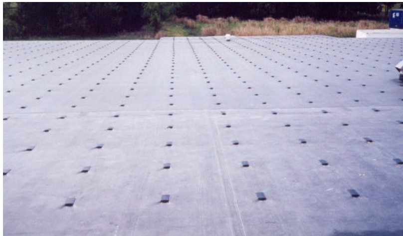
Black EPDM – the industry's most proven membrane technology – is formulated to slightly gray over time, actually increasing its solar reflectance capabilities as it ages.
